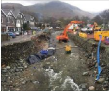
Glenridding village river channel blocked by boulders
